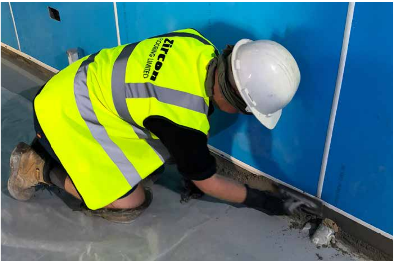
Installing cove detail
